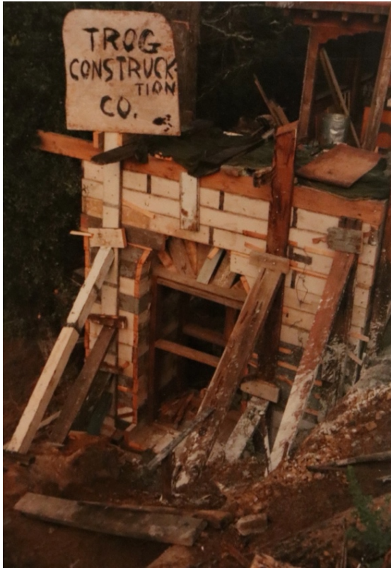
Figure 12. Woodshed Addition under construction, c. 1984. Photo Courtesy Susan Shannon.
