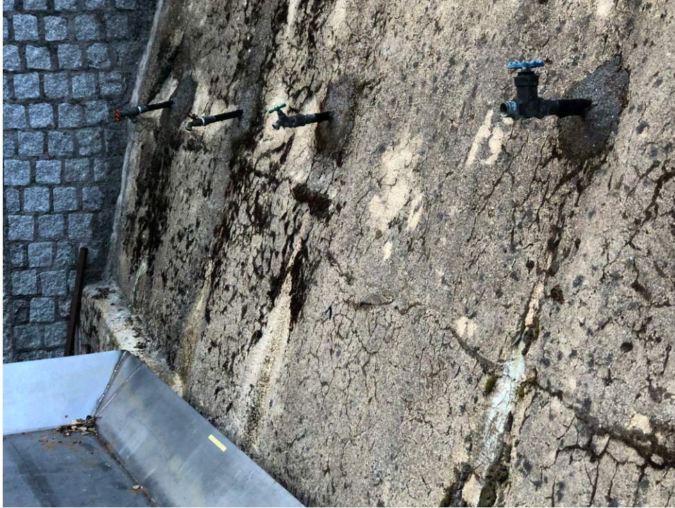
Figure 14. Graywater infrastructure. Spigots from separate garden terraces.
